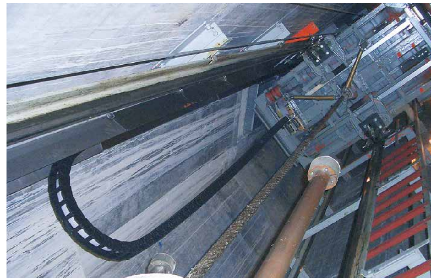
E2/000 - robust energy supply even with constant air draught and the resulting pendulum movements in this 160m lift for the Post Tower, Bonn
