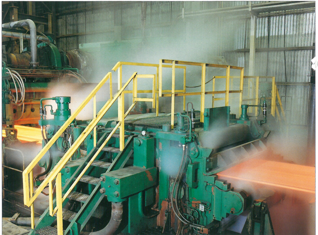
Descaler in front of a rolling mill of a thin slab casting mill
