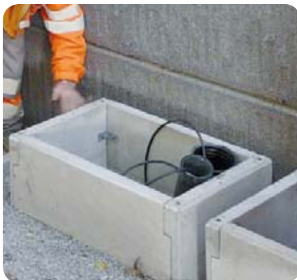
with suitable concrete slab
