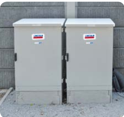
Outdoor pump cabinet 800 x 500 x 1200 mm
