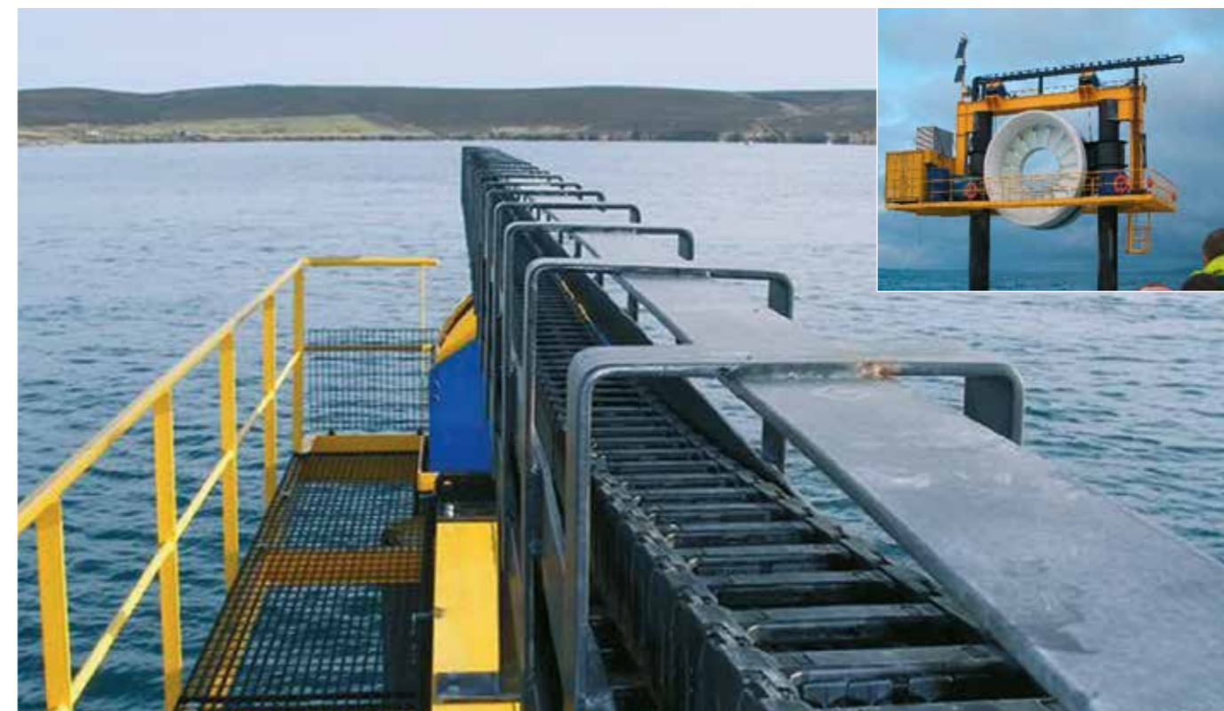
The maintenance-free series 4040HD protects the igus® chainflex® motor and signal cables during the lifting and lowering movements of this tidal turbine and protects them against the aggressive ambient conditions. 20m vertical movement above and below water
