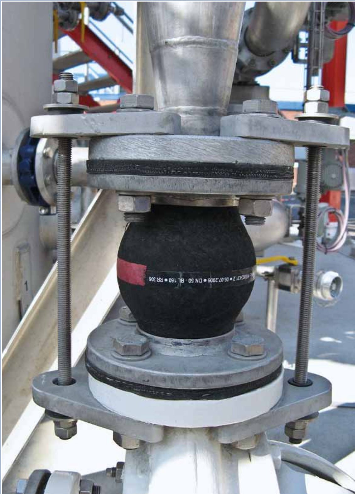
Lateral expansion joint, type U110R on the pump pressure side in a paper mill NB 50, 10 bar
