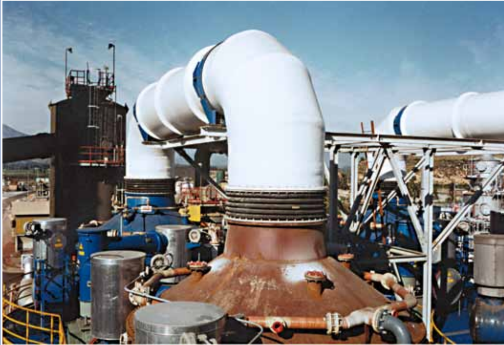
Universal expansion joint, type U152A with PTFE lining in a GFK pipe in a copper mill NB 2000, -0.17 bar, Earthquake movements all sides \pm 150 mm
