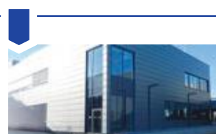
Opening of the ultra-modern Development and Technology Center in Metzingen
