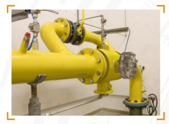
Unlike the classical method of installation in the pipeline, with the OEV the injection nozzle is installed directly into the ball valve.
