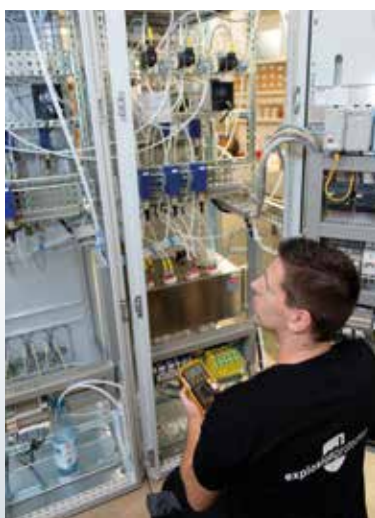
Calibration of an ACOM system
