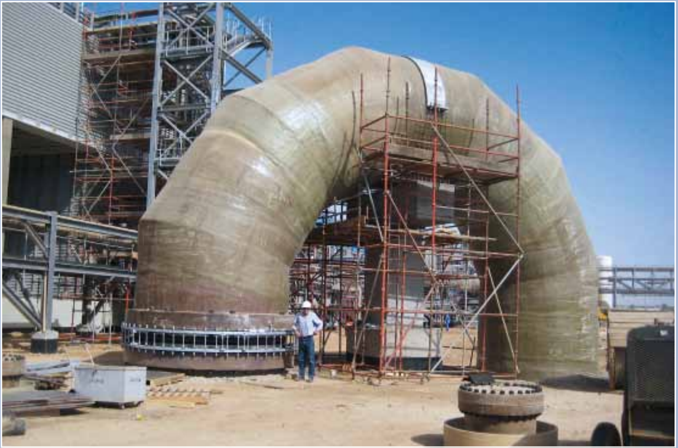
Type U110M lateral expansion joint in a desalination plant NB 3600, 8 bar, 90°C
