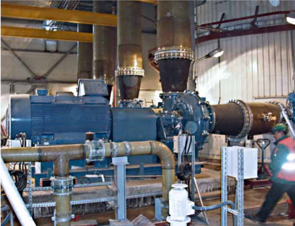
Universal expansion joints, type U300A-konz. on the pumps of a desulphurisation plant discharge side: NB 900 / NB 600, 4.5 bar, suction side: NB 900 / NB 700, 4.5 bar
