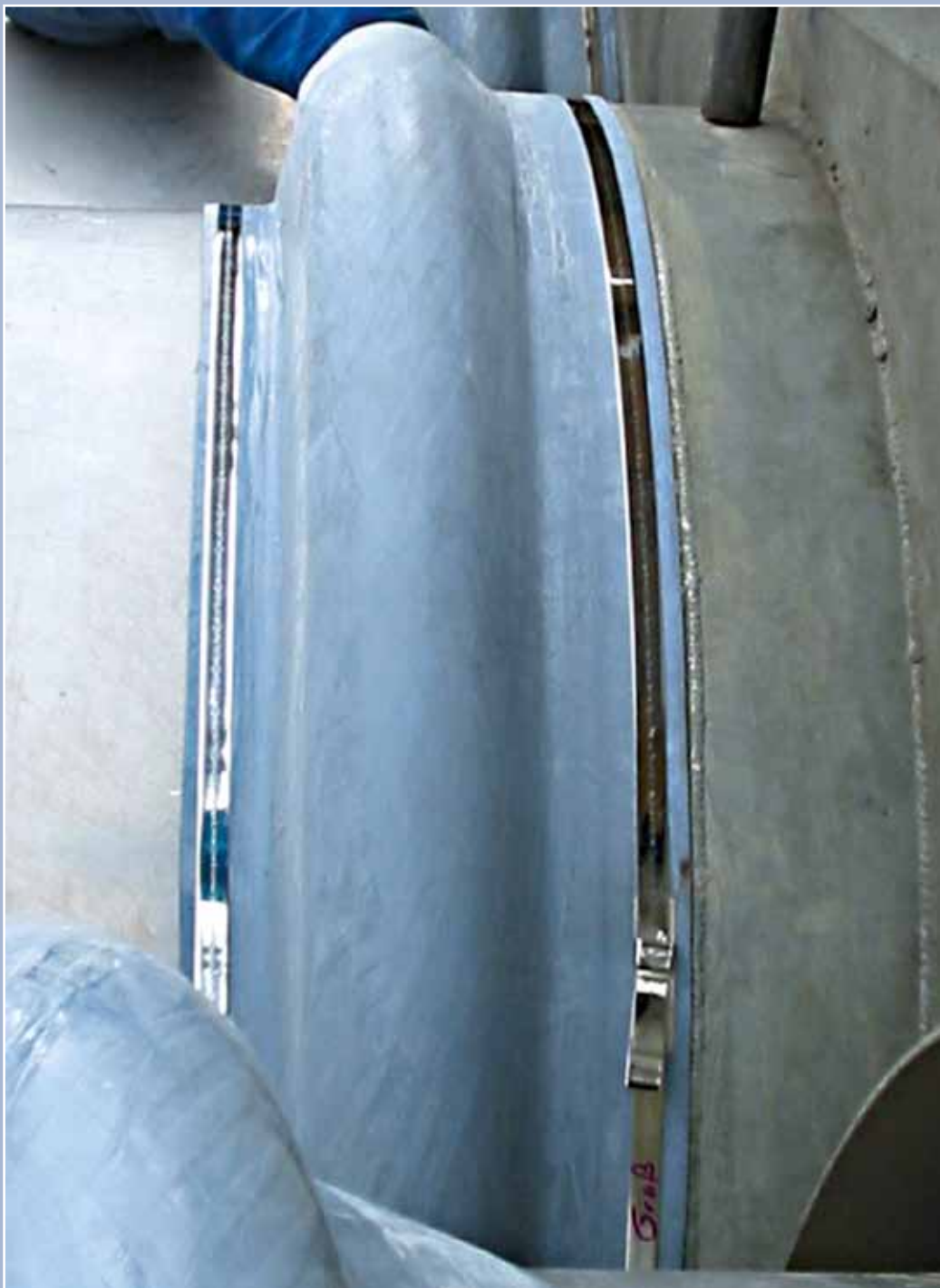
Universal expansion joint, type B310 as a drum connection NB 900 / NB 650, 0.1 bar
