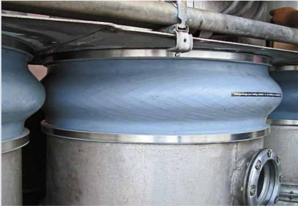
Universal expansion joint, type B110 in ventilation ducts NB 800, 0.15 bar
