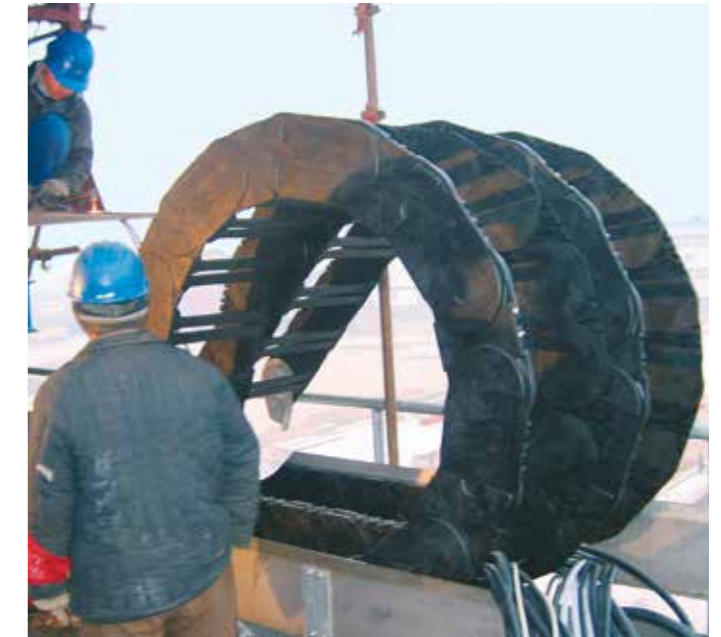
Assembly of an E4 e-chain® series 800 in a steel guide trough
